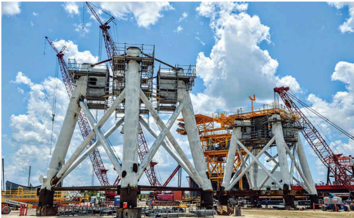
For an offshore project in Rhode Island, turbine supports were designed, fabricated and installed by Louisiana oil-and-gas firms.
